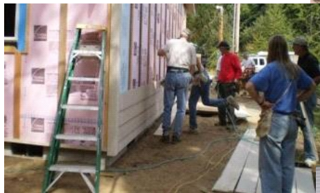
HFH Volunteers pitch in to install siding
